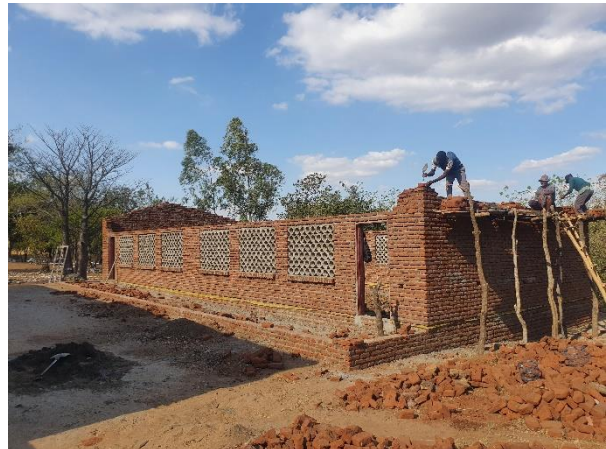
Figure 2: New School block
