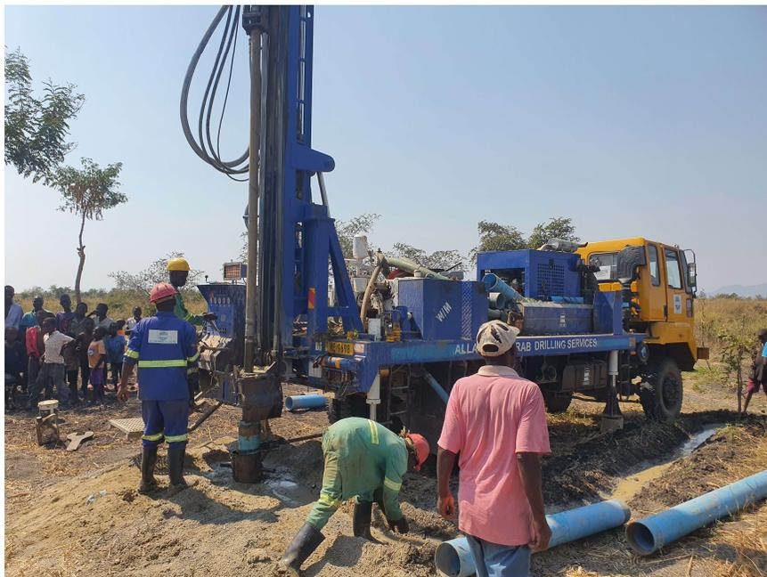
*Left- Drilling in progress at Lundu for the installation of the new pump*
